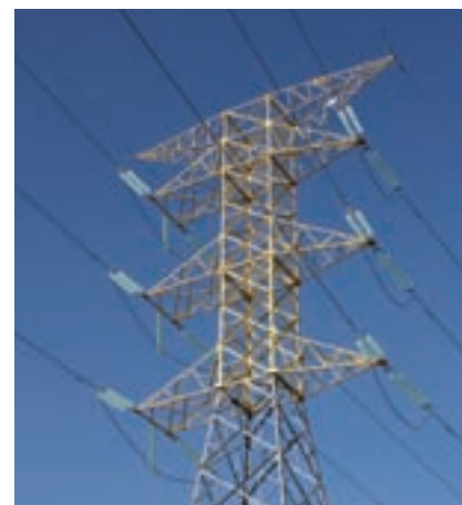
Figure 56 Due to its high electrical conductivity and low density aluminium is used to transmit electricity through overhead power lines
