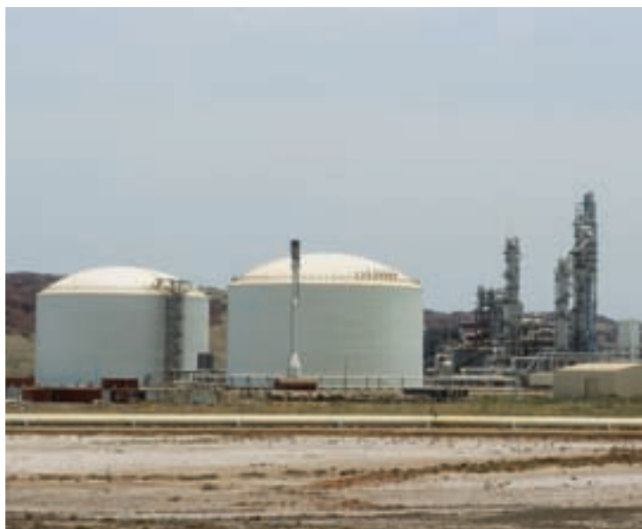
Figure 11 An ammonia production plant
