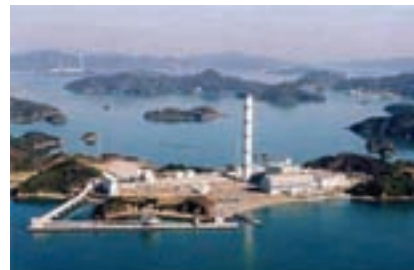
Figure 1 A pressurized fluidized bed combustion (PFBC) plant in Japan
