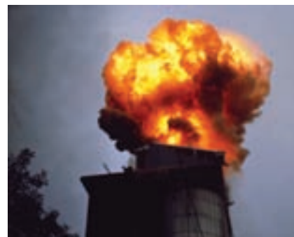
Figure 11 Dust explosion in a grain silo
