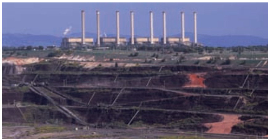
Figure 10 A coal-burning power station in Australia. In addition to contributing to global warming by emitting carbon dioxide, coal-fired power stations also emit sulfur dioxide.
